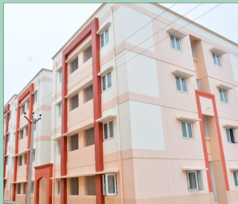
AHP Project Tamilnadu
